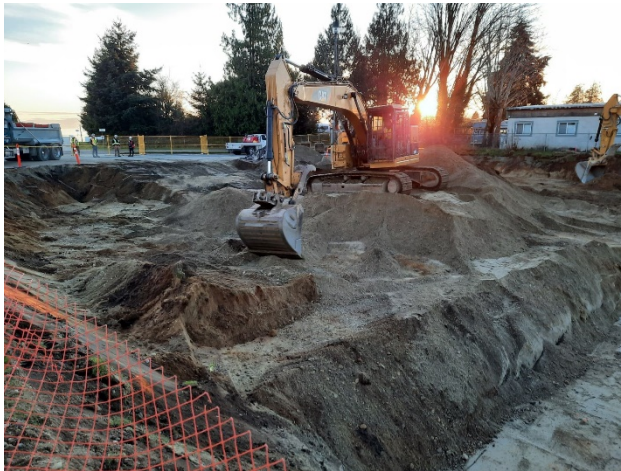
Excavation activities on December 4, 2020.
